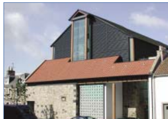
New development using modern and historic materials, Byre Theatre, St Andrews
