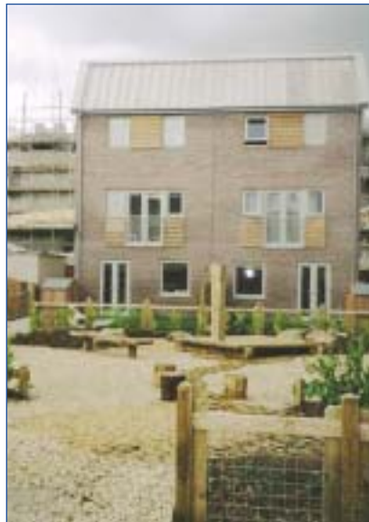
New development at Gateshead: development facing onto communal public space
